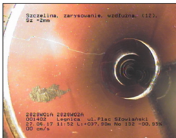
Foto 132 Video: CD1 Stan BAB A A 37,90 m 12 o'clock
